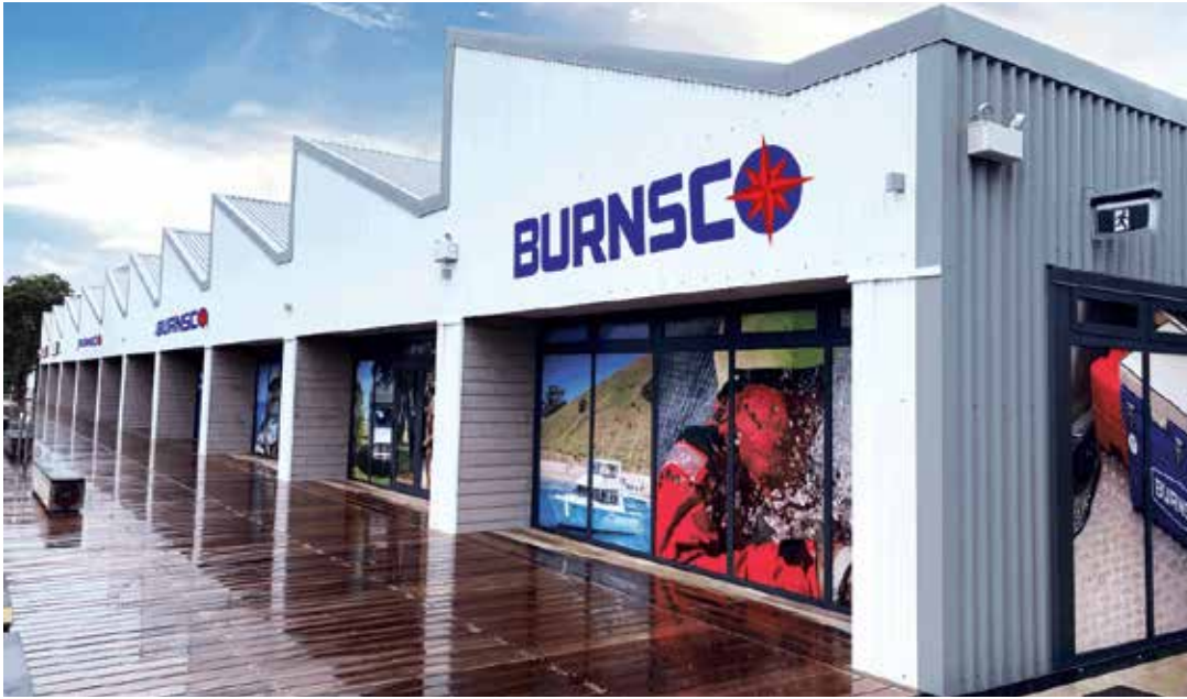
Burnsco's new Westhaven, Auckland store is now open for business.
