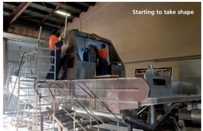
The hull under construction
